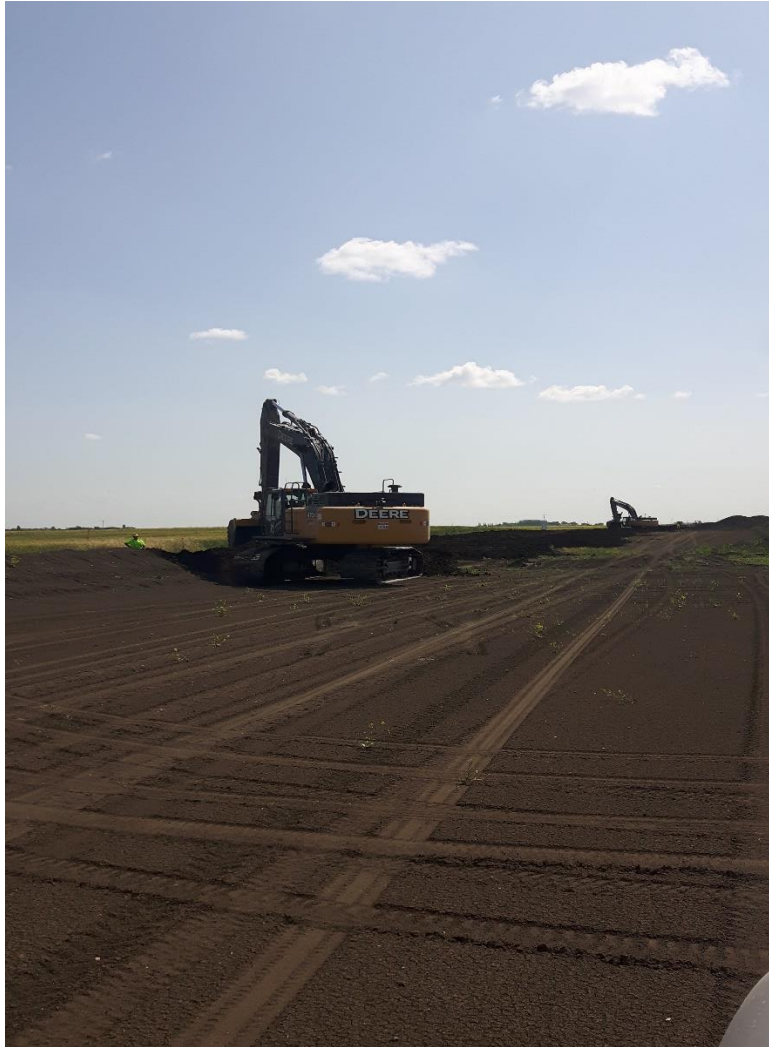
Machine Clean Up Crew de-compacting soil.
