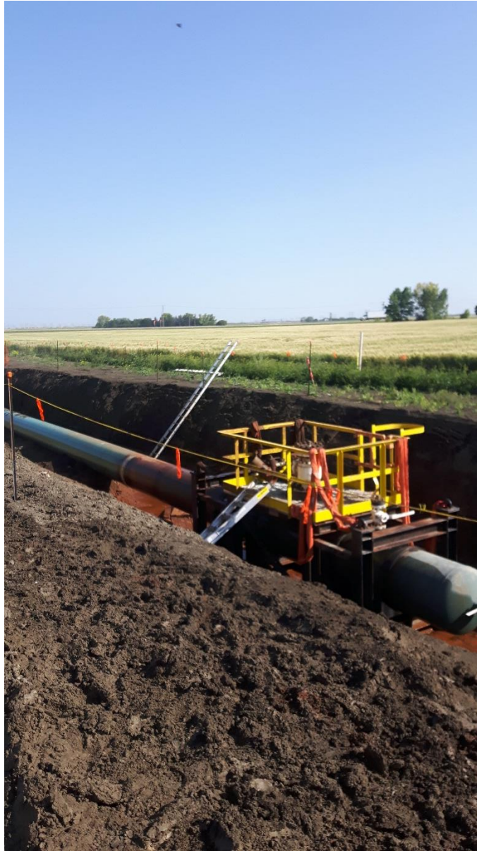
Test head welded on.
