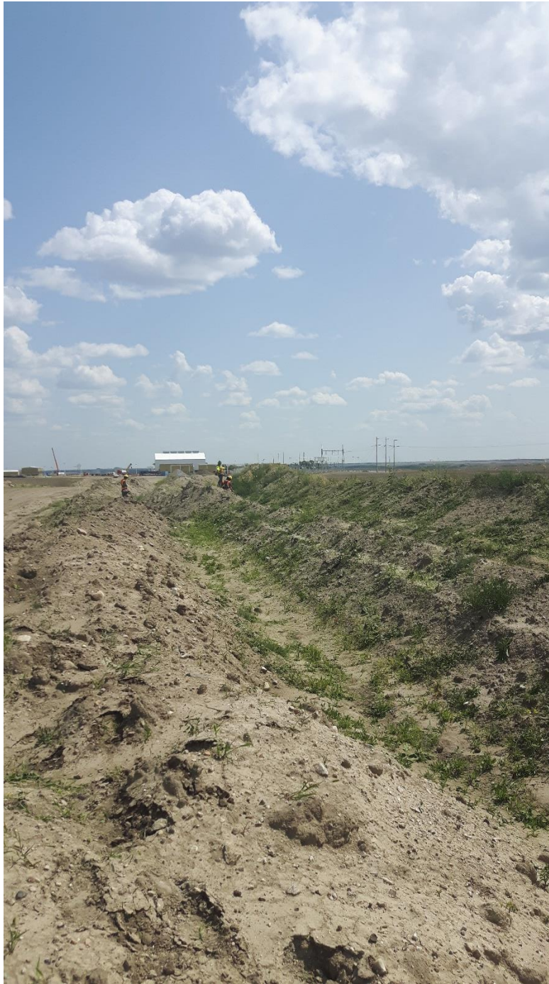
Trimming Weeds in Organic No Spray Zone on Topsoil and Subsoil.
